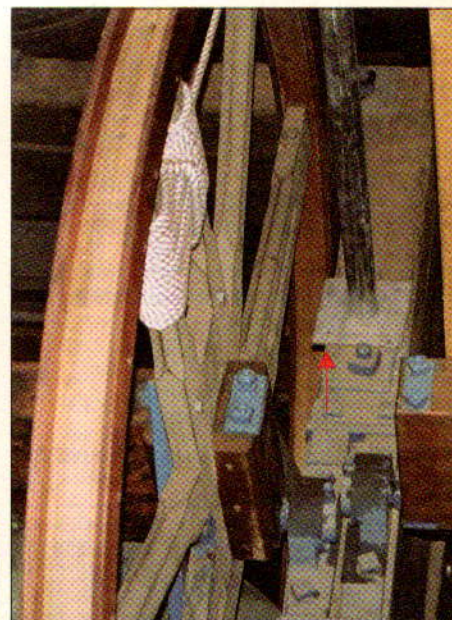
Too close for comfort? A precariously placed scaffolding pole Photo PLC
