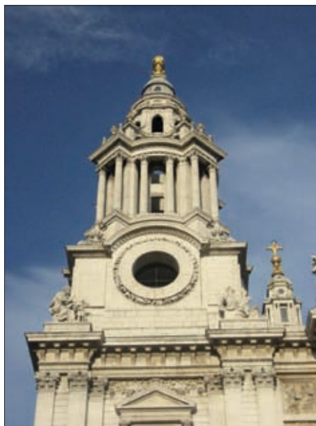
The north west tower which houses the 62cwt Taylor twelve (Photo by the Editor)
